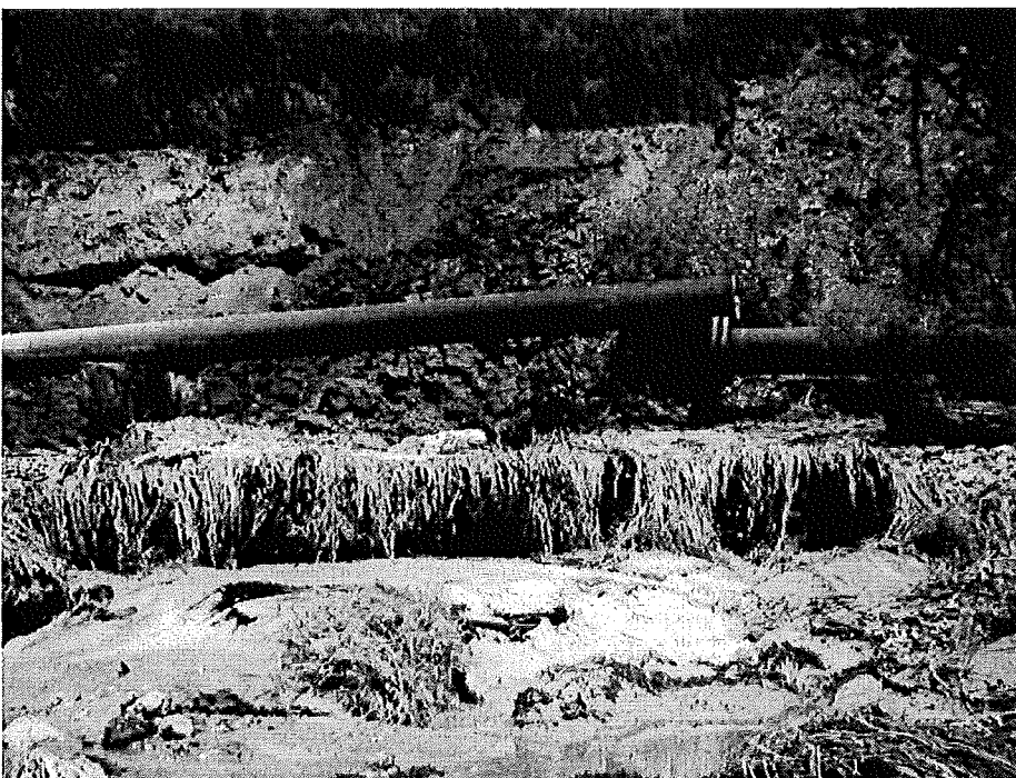
Picture 10: Liquid discharging into Bayou Casotte at site#2 Concrete Ditch/Break continued. 081913
