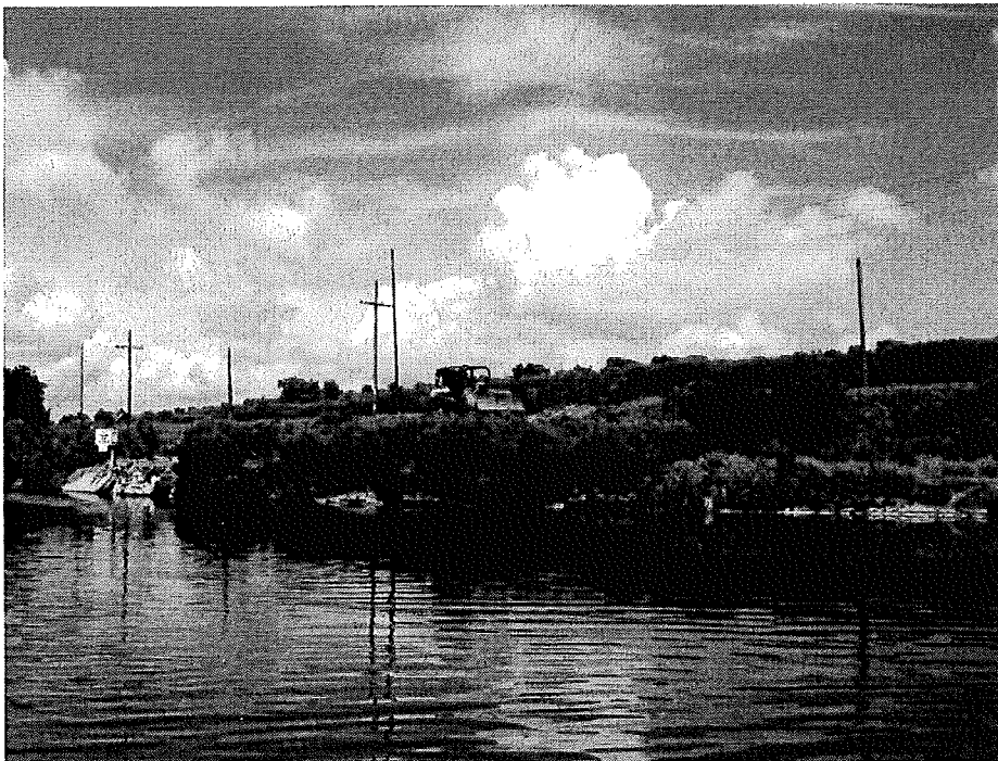
Picture 4: At site#2 Concrete Ditch/Break. Heavy machinery moving dirt to repair dike. 081913
