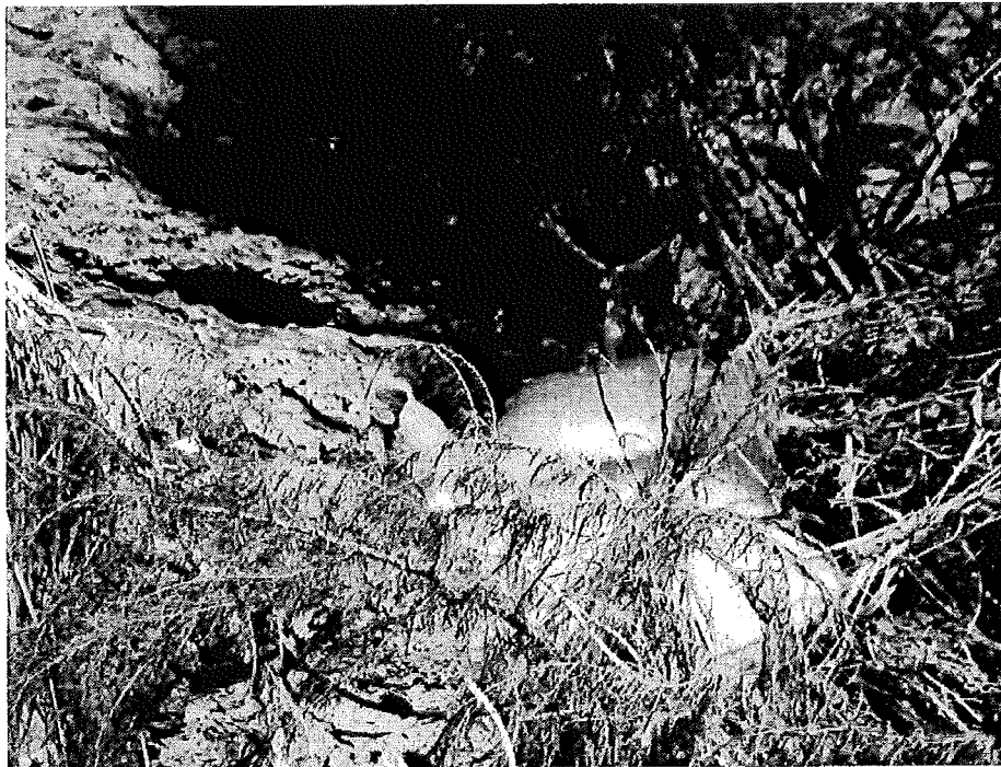
Picture 8: Liquid discharging into Bayou Casotte at site#2 Concrete Ditch/Break continued. 081913
