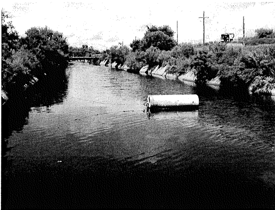
Picture 5: Site#2 Concrete Ditch/Break 081913
