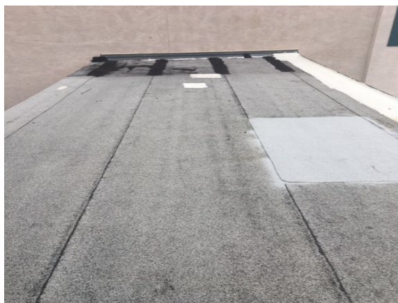
Patched damaged roof area
