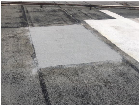
Installed modified patch
