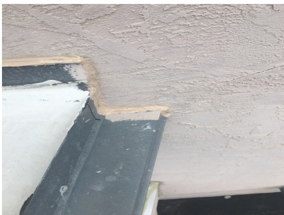
Cleaned and sealed metal wall flashing
