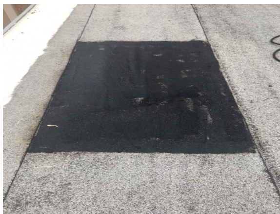
Patched damaged roof area
